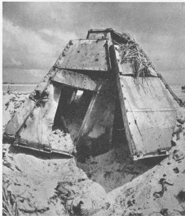
Figure 111. Steel pillbox on Tarawa.
