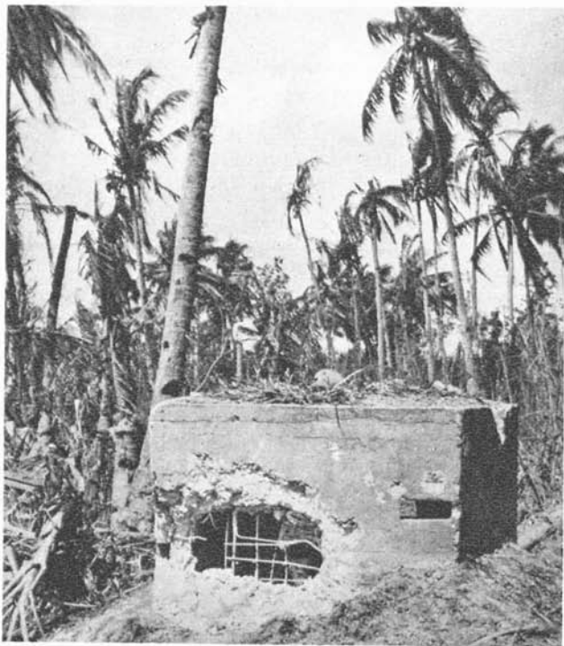
Figure 109. Concrete pillbox on Guam.
