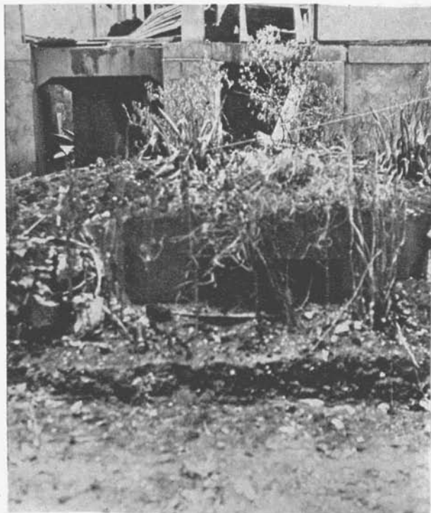
Figure 110. Cleverly concealed concrete pillbox under a Saipan building.
