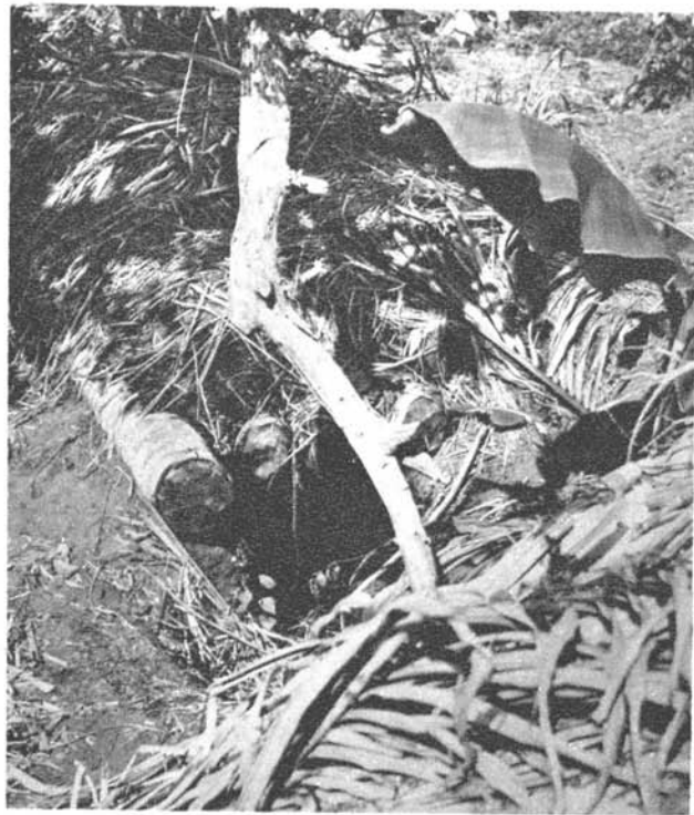
Figure 105. A well-built and concealed pillbox.
