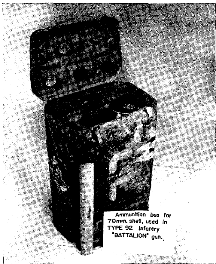
Figure 144.—Metal carrying case for 70-mm high-explosive shells (five complete rounds).
